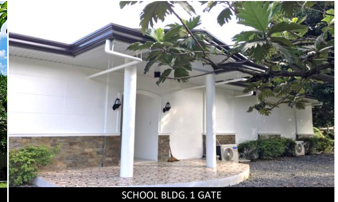
SCHOOL BLDG. 1 GATE
